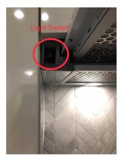
The lamp switch is located on the left side of the hood.
