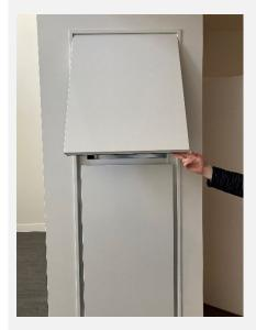
In some applicable townhomes and live work homes, there is a thermal recovery unit (ERV) that draws clean, fresh air into the home. ERV's transfer heat and moisture through incoming and outgoing airstreams.
