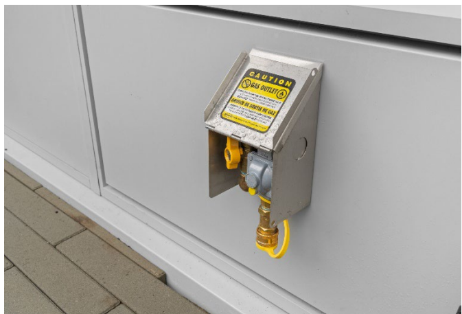
Exterior gas shut off in the "on" position.
