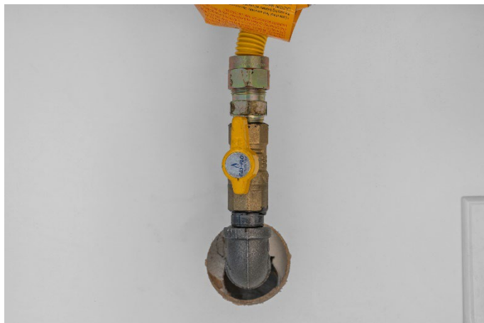
Gas shut off in the "on" position.
