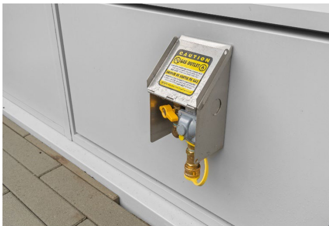
Exterior gas shut off in the "off" position.
