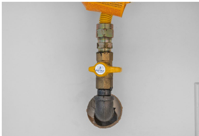
Gas shut off in the "off" position.
