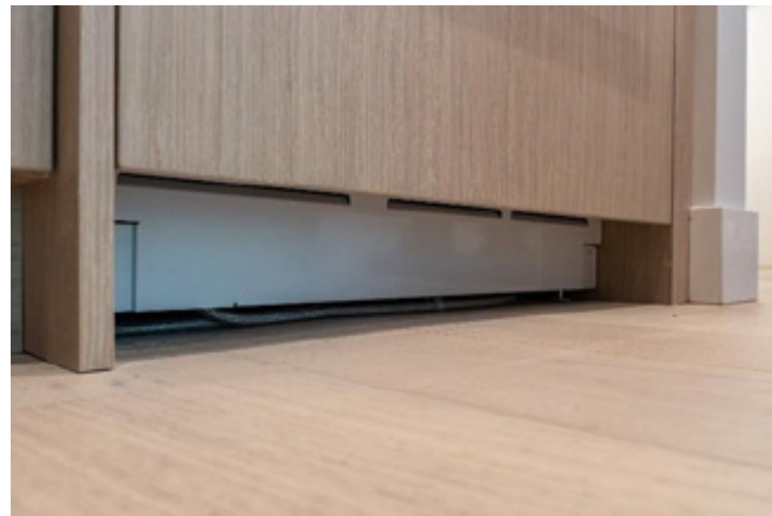
Remove the toe kick panel.
