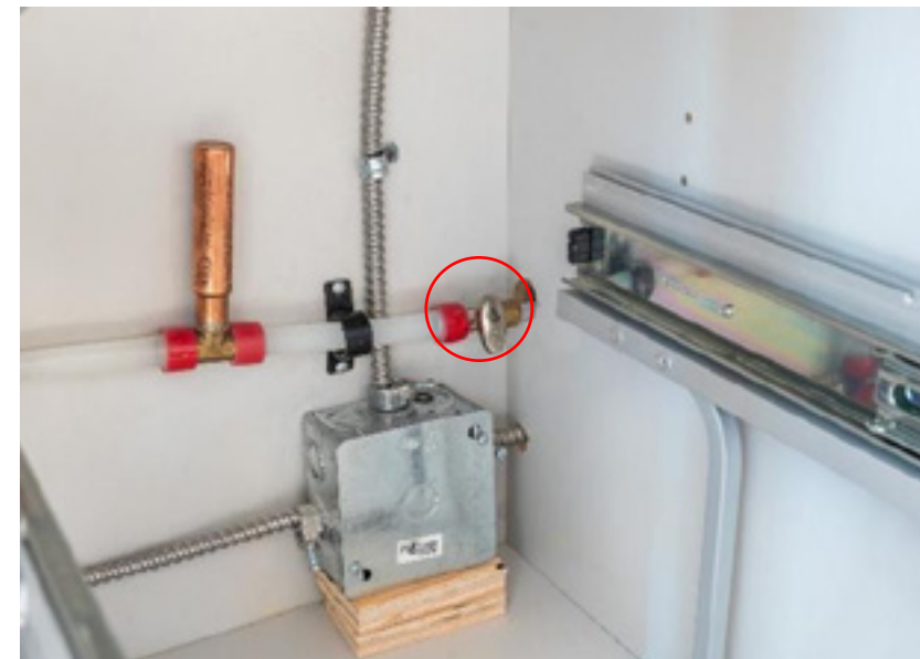
Be mindful that your dishwasher water shut off may be behind the rolling waste bins.
