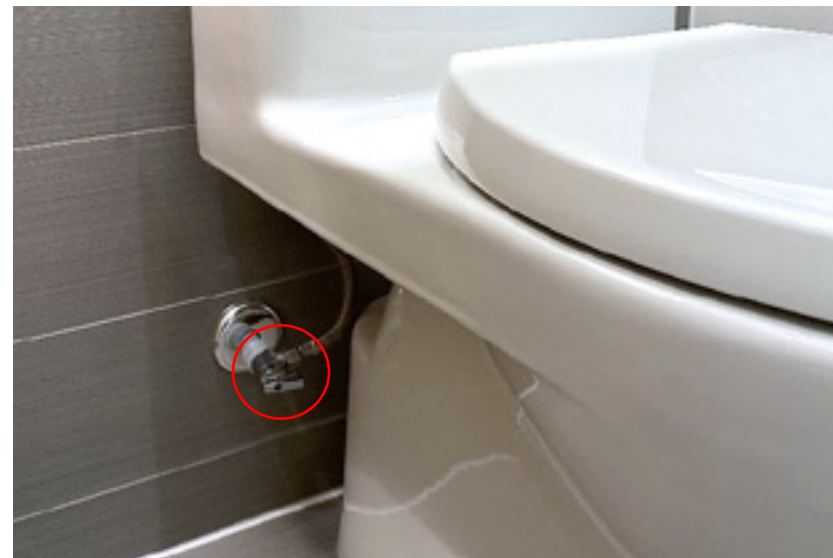
Toilet shut off behind the toilet.
