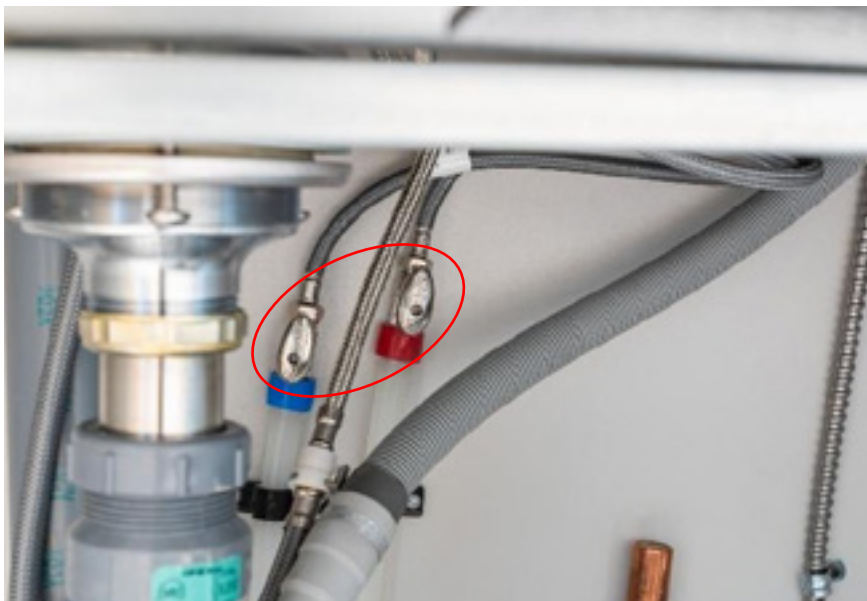
Faucet shut offs below kitchen sink.
