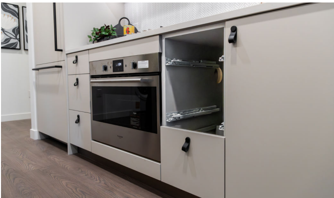
Gas shut off location for the cooktop is behind the cabinet drawer.
